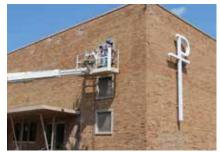
Replacement of broken bricks and tuck pointing
