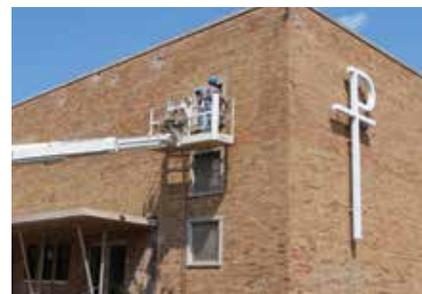
Replacement of broken bricks and tuck pointing
